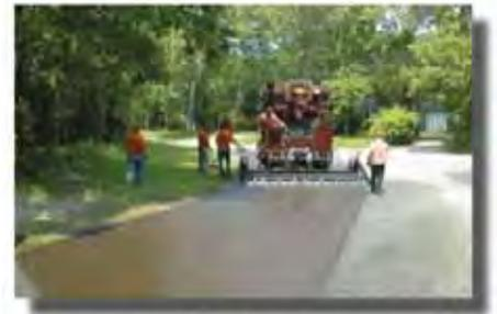
*Application of skid-resistant pavement surface in curve.*
