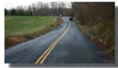
*Centerline for No Passing on horizontal curve.*
