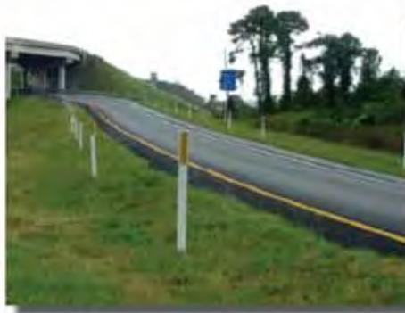
*Post delineators installed on a ramp.*
