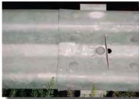
*Installation of reflectors on W-beam guardrail.*
