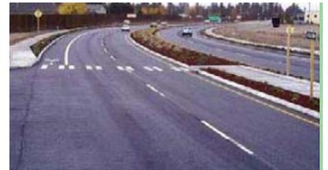
Crosswalk safety can be enhanced by proper location, high visibility markings, illumination, signing, advance stop bars, median islands, curb extensions, and signals.
