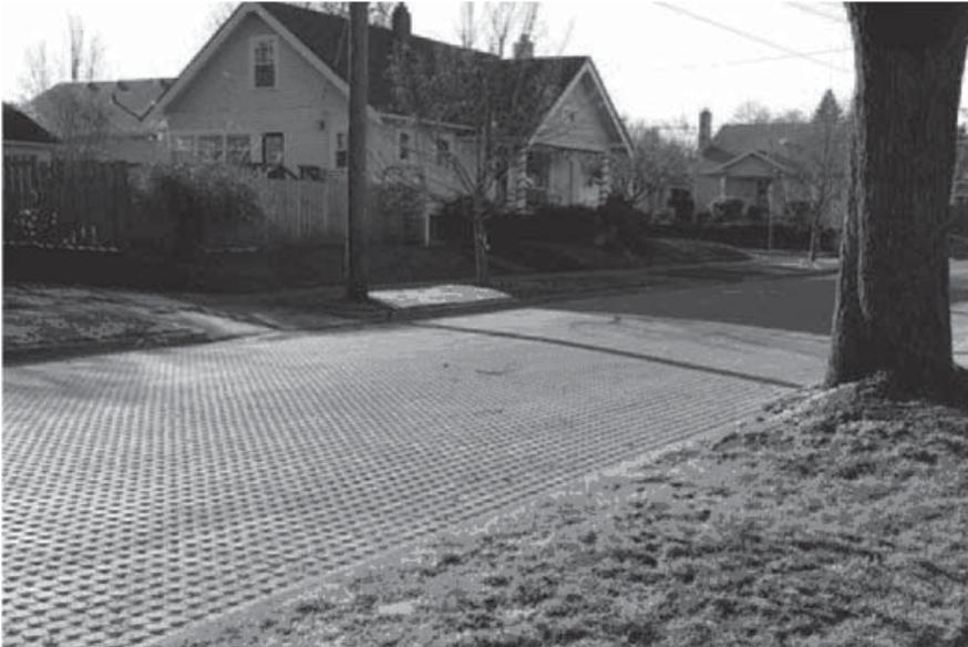
Interlocking concrete pavements not only provide a serviceable pavement surface but also can be designed to serve as a storm water drainage system. Several cities have recently taken advantage of this potential by choosing to use permeable interlocking concrete pavements (PICP).
