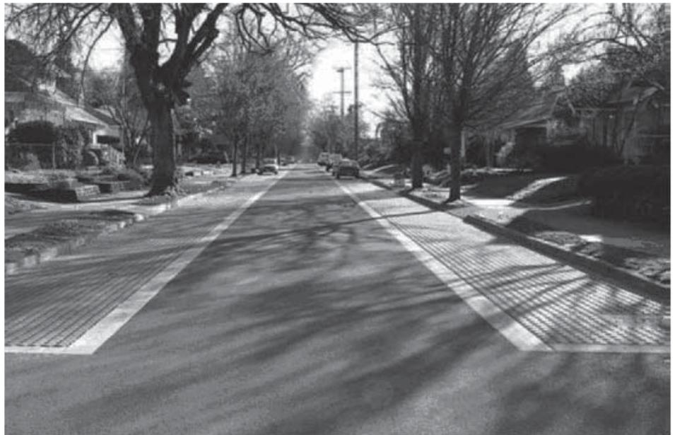
The permeable pavers receive runoff into an open-grade aggregate base, or “drainage blanket,” that extends under the asphalt across the entire street. This boosts water storage and infiltration capacity.
