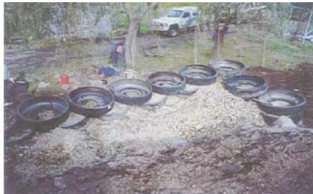
*Photo 1 Looking Down on Tire Placement & Granular Backfill.*
