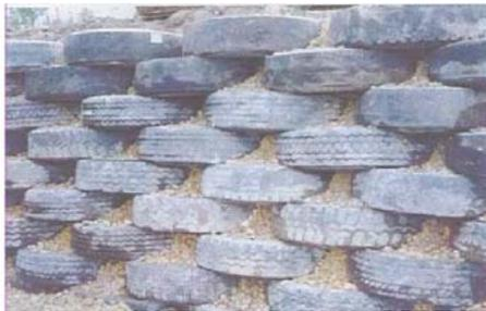
*Photo 2 Looking at Face of Wall Showing Layering of Tires.*
