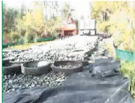
Photo 4 Installation of Roadway Stabilization over Soft Ground.
