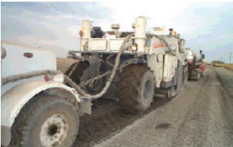
As the recycler pulverizes the road, the hot asphalt is foamed by the addition of a small (2-3% to the volume of asphalt) amount of water. The foamed asphalt at-
