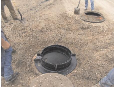
**The initial manhole cover assembly base is installed.**
