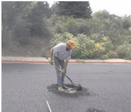
**Excess asphalt is removed; the surface around the cover is compacted.**
